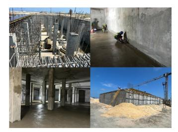
Xypex Concentrate was applied to ensure permanent and integral waterproofing, forming a crystalline structure within the concrete that prevents water infiltration and enhances durability.
